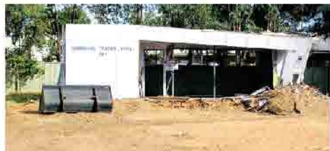
Trades Hall demolished
